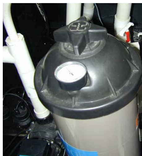
Filter locking nut ( Fig N (a) )
