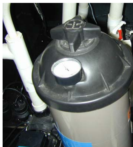
Filter locking nut ( Fig N (a) )
