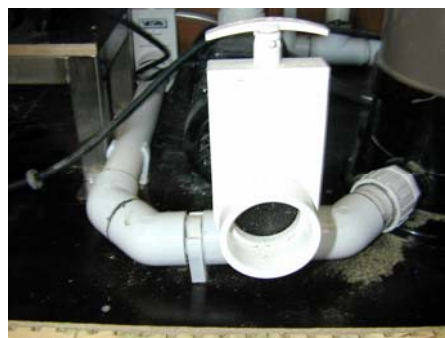
Pool Section Drain (Fig N)
