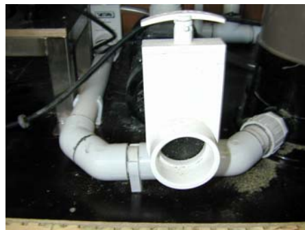
Pool Section Drain (Fig N)
